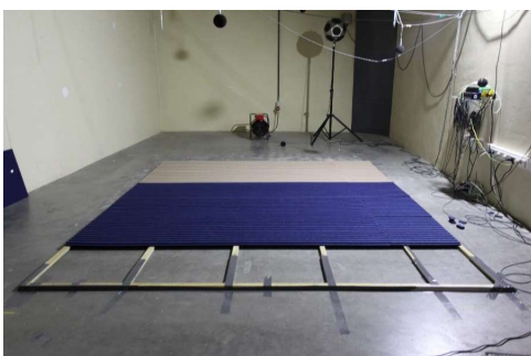
photo : Test n° 23 : during placement of the panels on the empty frame
