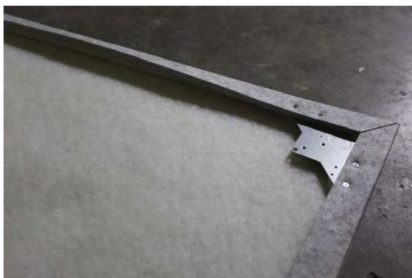
photographs : back of the ceiling island, filled with acoustic fleece
